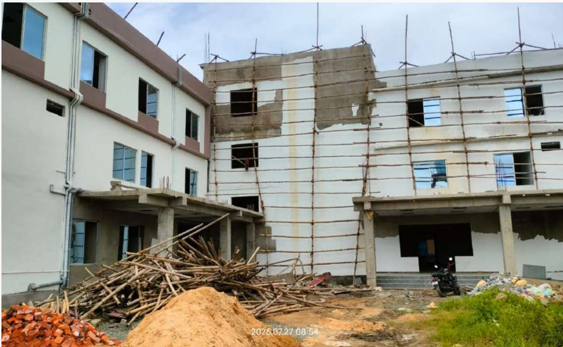
New Construction: 50 bedded " Critical Care Block" at District Hospital Thoubal under PM-ABHIM
